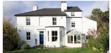
39 St James Road, Edgbaston
