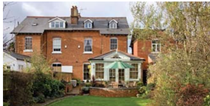
66 Wheelays Road, Edgbaston
