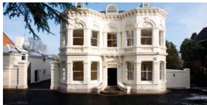
10 Farquhar Road, Edgbaston
