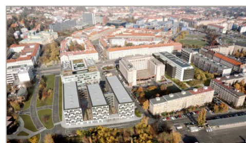
BPD development launched reconstruction of Telehouse in Prague 6. The project will offer approx. 20 000 sqm of office space.
