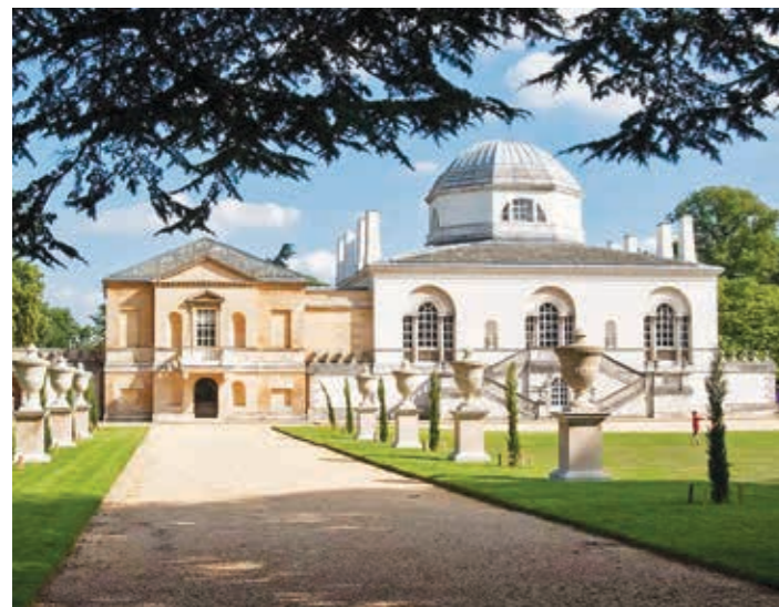
1. CHISWICK HOUSE Designed by the Earl of Burlington in 1729, Chiswick House is a magnificent Grade I-listed villa set in landscaped gardens. Inspired by the buildings of ancient Rome, it is one of Britain's best examples of Neo-Palladian architecture.
