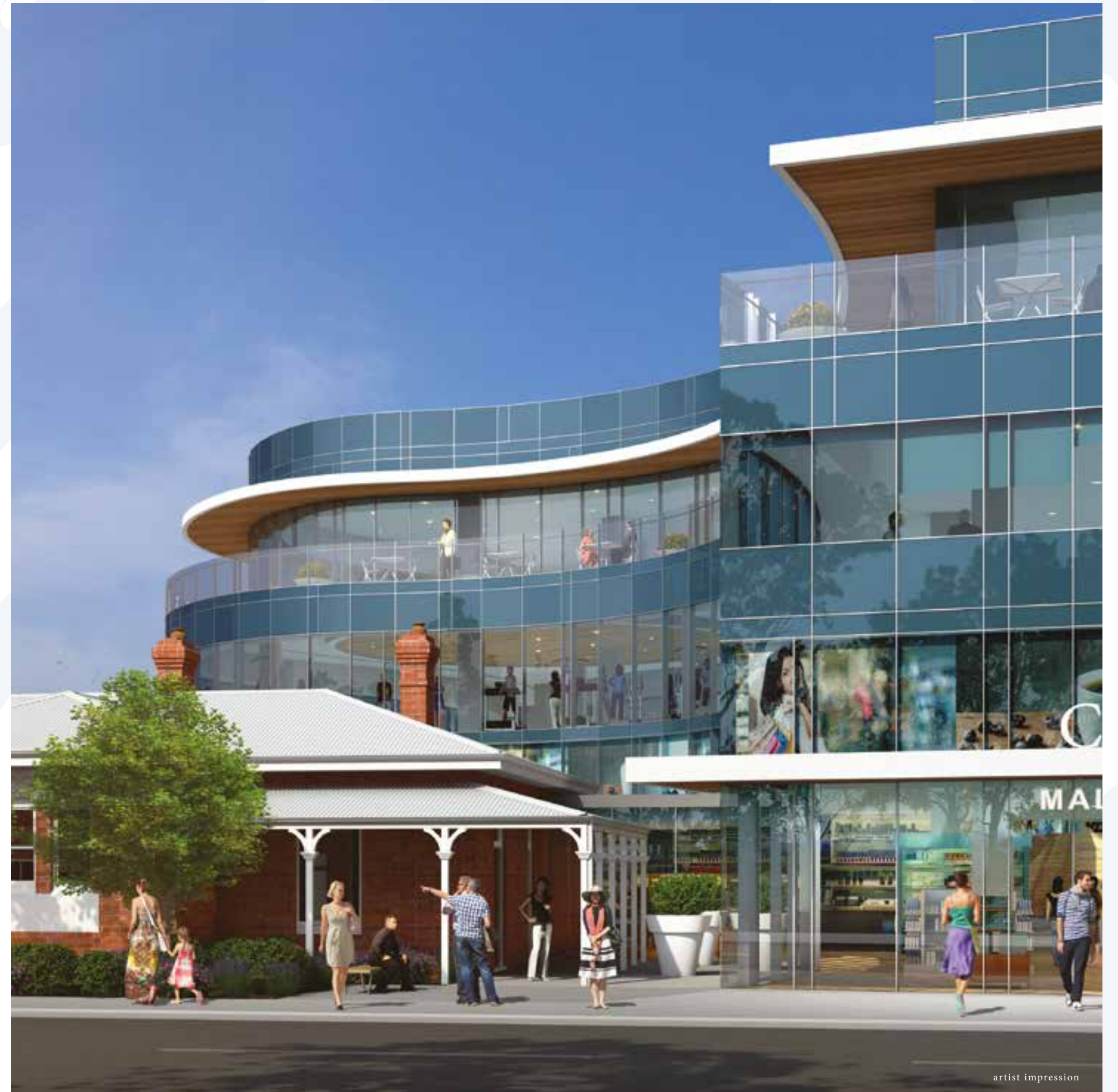
SOUTH PERTH POST OFFICE
